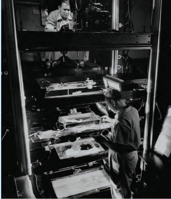
From left to right: Disney's four-layer camera, an invention of the Disney studios, photographs four celluloid drawings together, giving an illusion of depth to cartoon action. Steamboat Willie was released in 1928.
